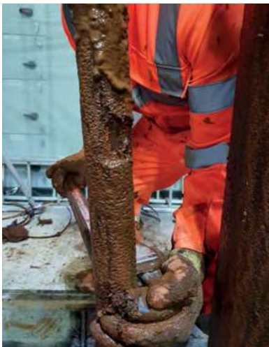
An example of typical iron bacteria residues on a pipe prior to treatment
